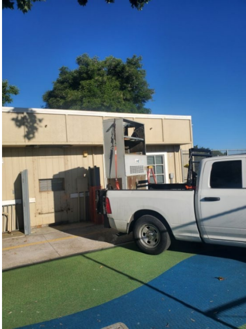
HVAC Install at Jane Addams
