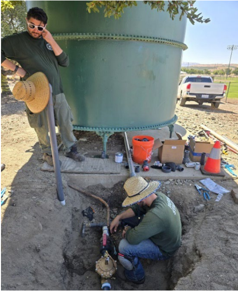
New Master Valve installation at Ernie Rodriguez
