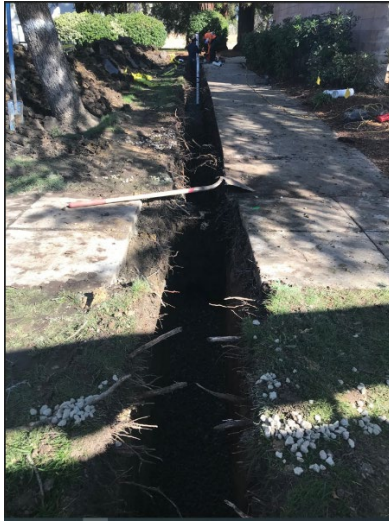
Trevano Road Sewer Project
