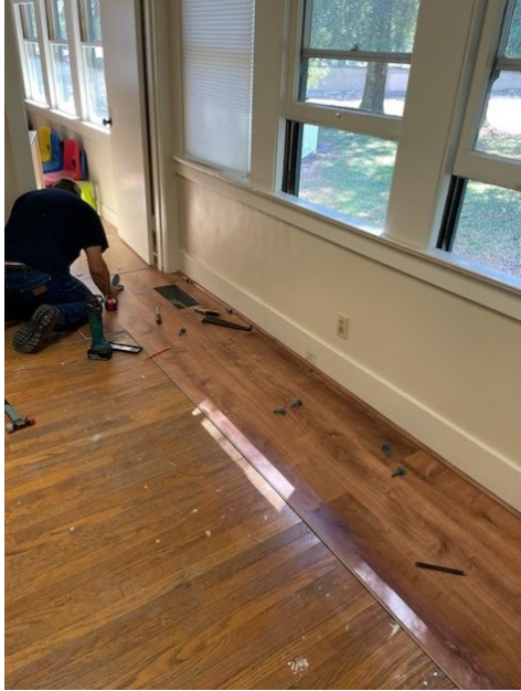
Flooring at Little House Preschool
