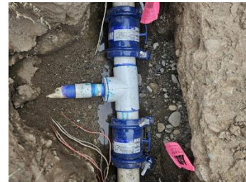
Ongoing irrigation repairs:
