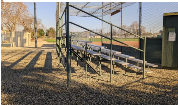
New Bleachers installed by Facilities Team.
